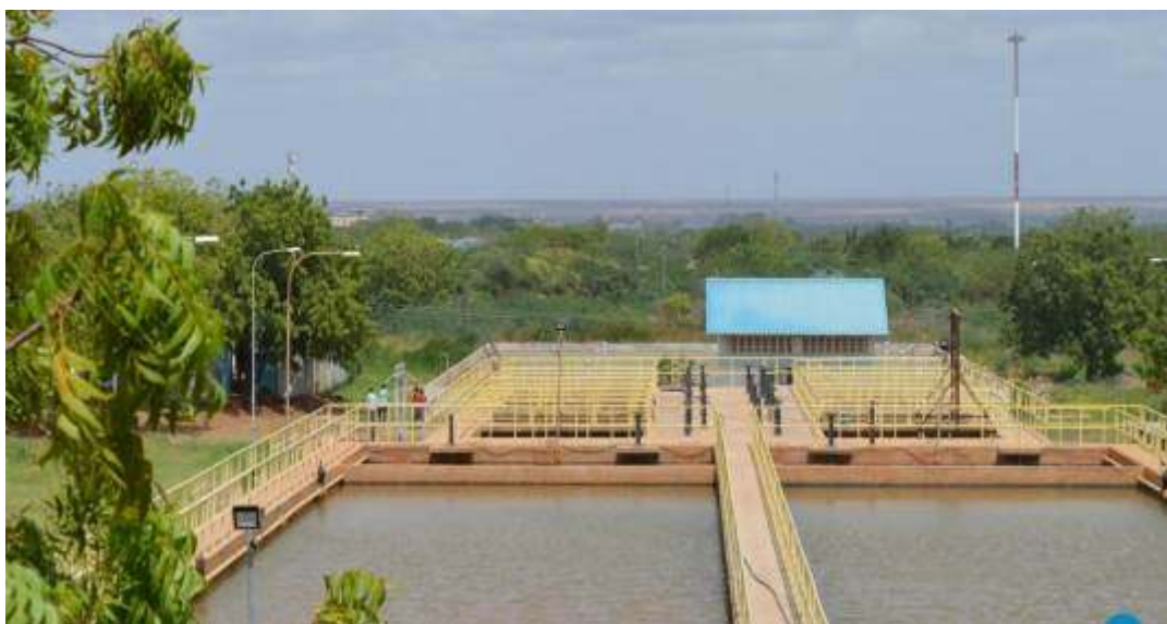
Plate 3: View of the water treatment works infrastructure by GAWASCO
